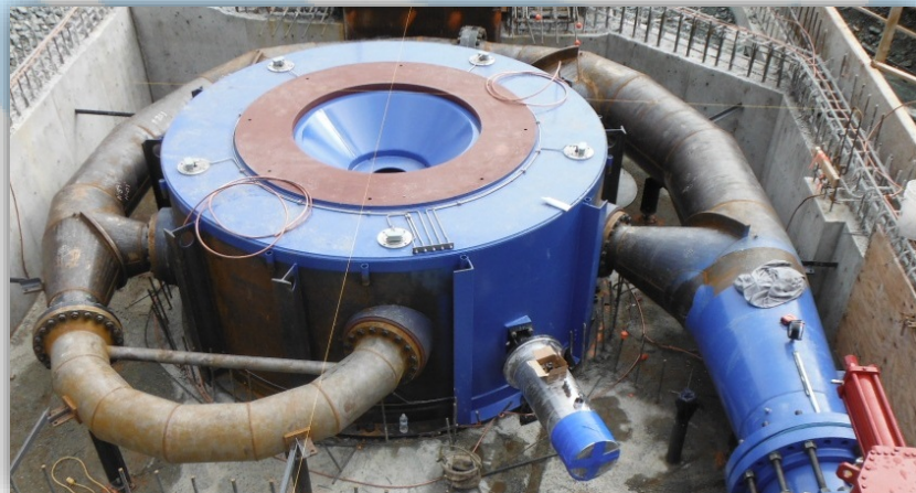
Figure 4: 4.3 meter diameter A572 steel housing and ANSI 300 Class water delivery system fabricated by Canyon
