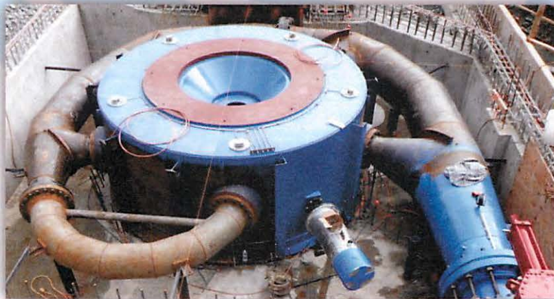
Figure 4: 4.3 meter diameter A572 steel housing and ANSI 300 Class water delivery system fabricated by Canyon
